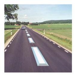
Figure 3: Three-dimensional markings
