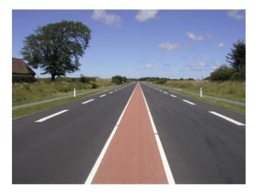
Figure 14: Red coloured central area flanked by reflectors.
