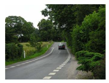
Figure 10: Transition from"2-1"rural road to the ordinary two-lane rural road with centre line ahead
