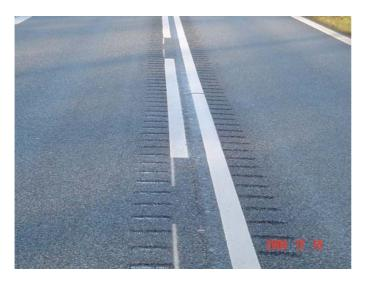
Figure 7: Rumbling marking along centre lines
