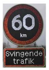
Figure 12: VMS sign showing temporary speed limit and warning for crossing traffic ahead.
