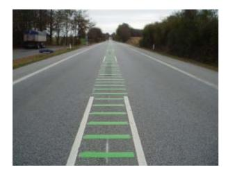
Figure 5: Centre line marking – design A.
