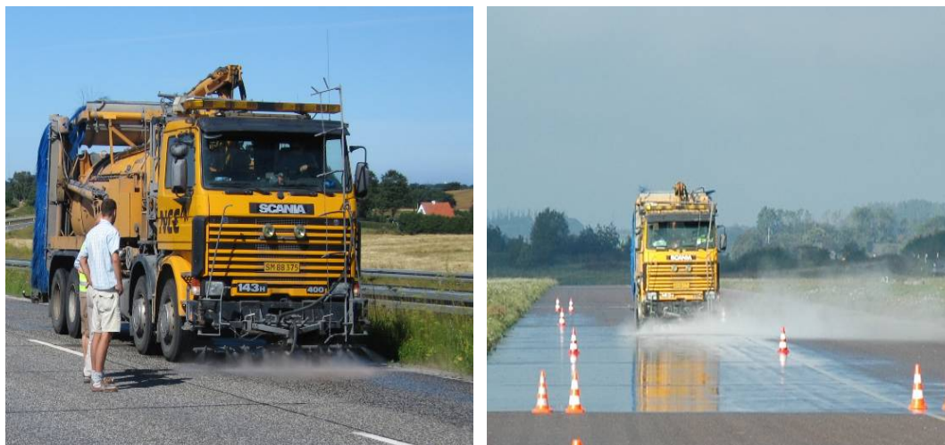
Figure 2.3 Roadway made wet using a water truck.
