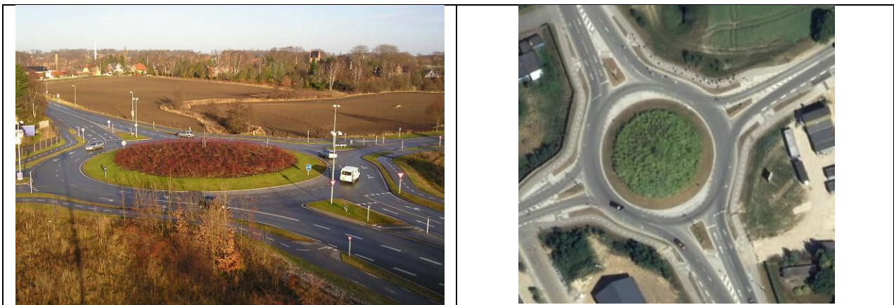
FIGURE 1. Typical 2-lane roundabout with separate cycle tracks outside the roundabout.
