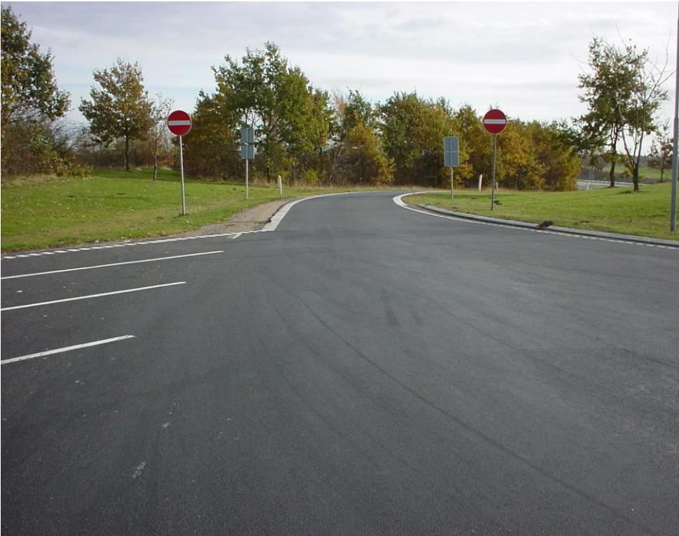
FIGURE 6: “Fish Trap Design Principle” that invites the driver to enter. But in this case it has been used wrongly because it is an exit that invites the driver to enter. Only enterings should be given this fish trap design while exits should be invisible or designed to give a “refuse” signal to the drivers
