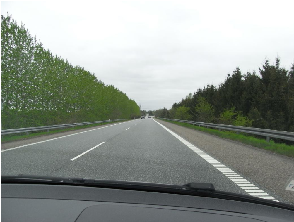
FIGURE 5: Photo example of Design B - wrong
