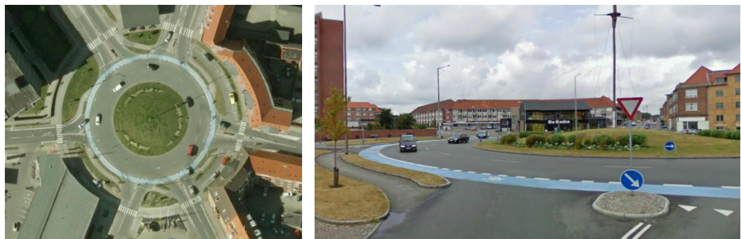
The roundabout at Frodesgade/Gl. Vardevej in Esbjerg.
