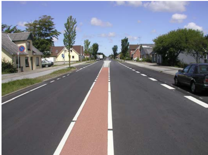
Figure 8.2: Small central islands have been added on sections going through the small town Harken.
