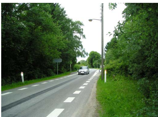
Figure 6.1: "2-1"- cross profile with one central driving lane
