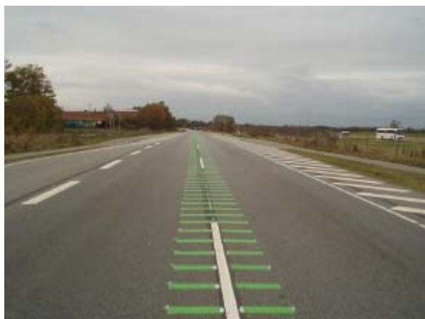
Figure 5.1b: Centre line marking – design B
