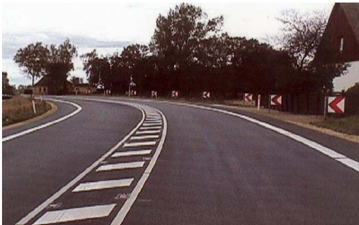
Figure 7.1: Chevrons in dangerous curves illuminate if speed is too high
