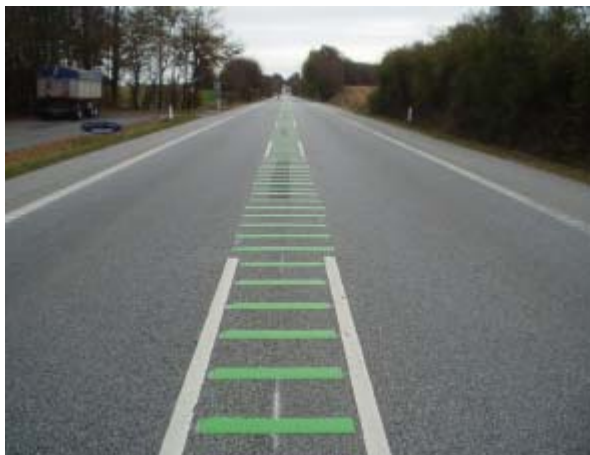
Figure 5.1a: Centre line marking – design A.
