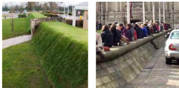
Figur 7.11 Udformning af vold til fysisk terrorsikring. Referencer Hostile vehicle guidelines for crowded places [5] og High Street Hospitality: Protective Security Considerations [6].
