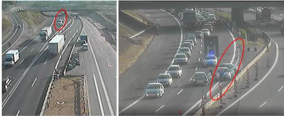
8 9 10 Figure 4 Example of a loss of left-hand lane taking the road users by surprise. The lane loss is 11 placed under a bridge in a curve just before a lateral displacement. Furthermore, the taper is very 12 short, notification of the lane loss is poor and the old edge line can be misleading the road users.
