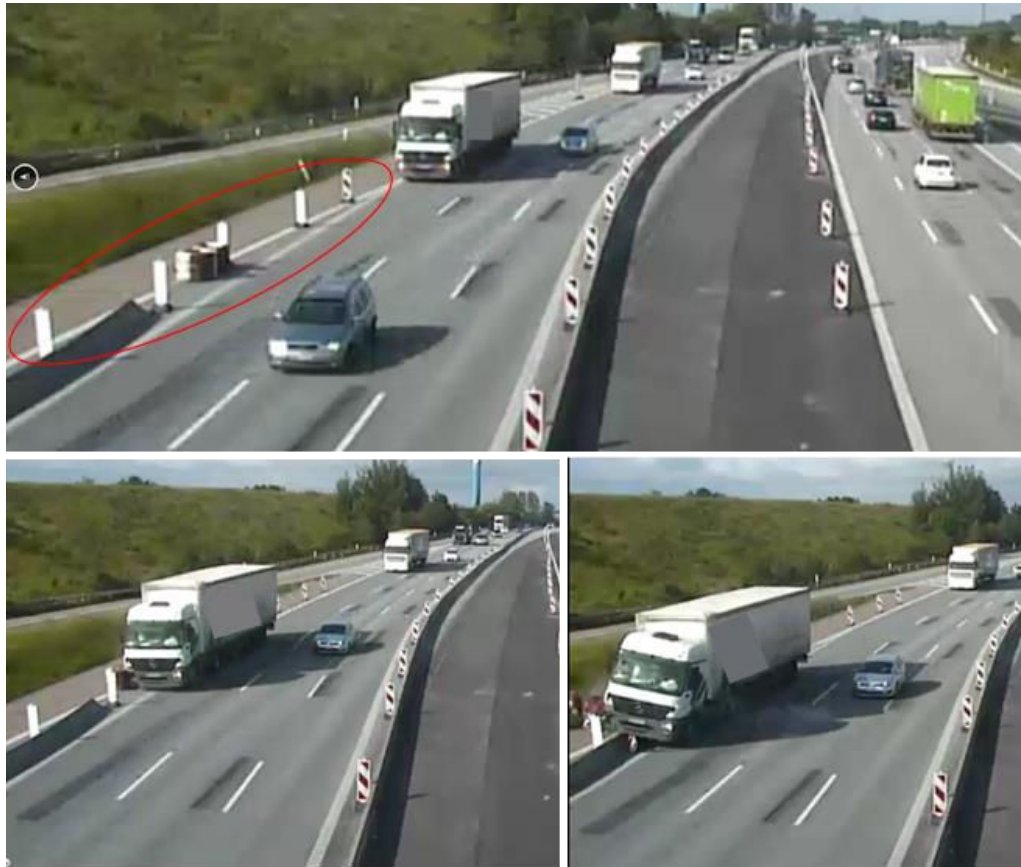
4 5 6 Figure 3 Example of old edge line and delineators misleading some road users. The driver of the 7 truck follows the old edge line and continues straight in the S-curve. 8
